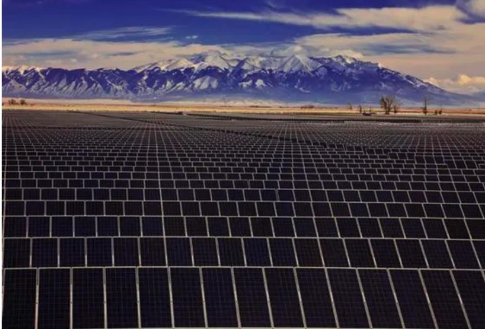
8.22 megawatts Capacity of the SunEdison Alamosa solar plant, above 1,652 Number of homes able to be powered by the plant in 2008
